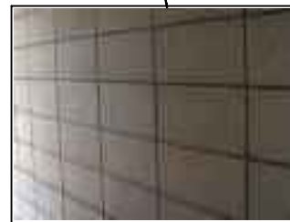
Masonry Polished concrete masonry.
